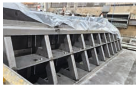
Support formwork for wall thicknesses up to 120 cm
