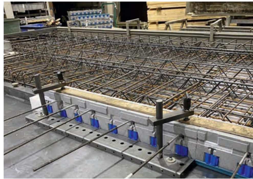
Adapter solution for thermal insulation elements for balcony connections
