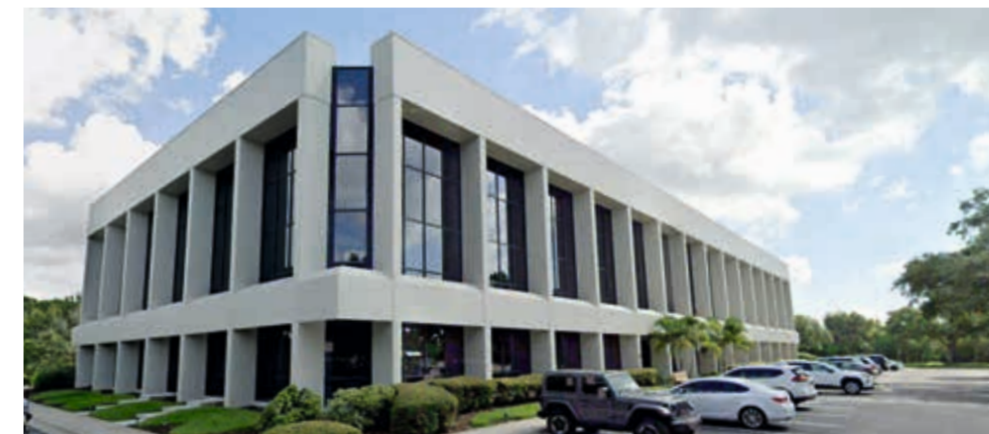
RATEC America has found a new home in this office building in St. Petersburg, FL
