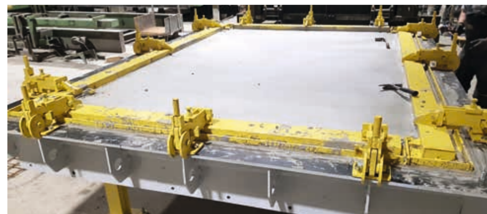
Roof mould for horizontal production
