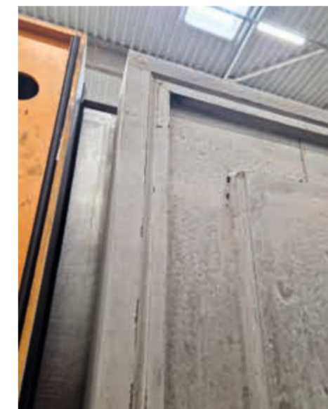
Finished roof element
