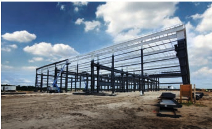
Summer 2020 – assembly of production halls 1 – 3
