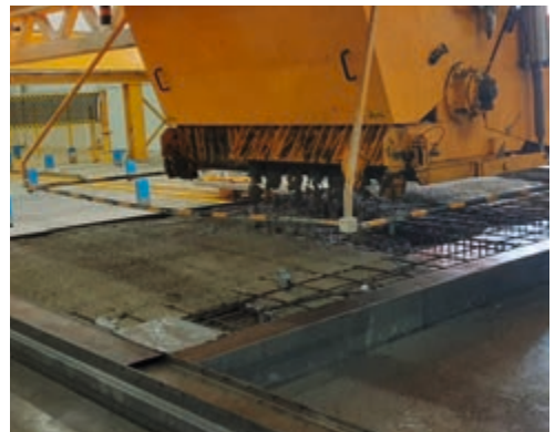
On-demand concrete supply
