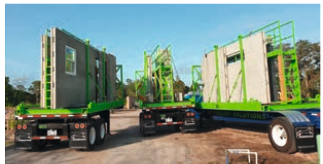
The handling in the outside area is done by a mobile gantry crane, which stores and retrieves the wall transport racks.
