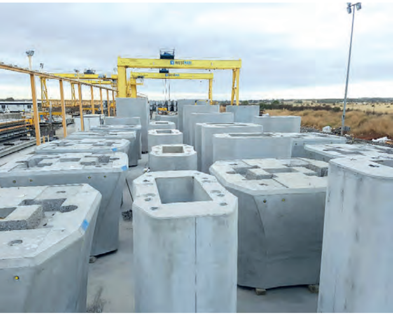
It was not possible to fill from above due to the diverse recesses in the upper face of elements.
