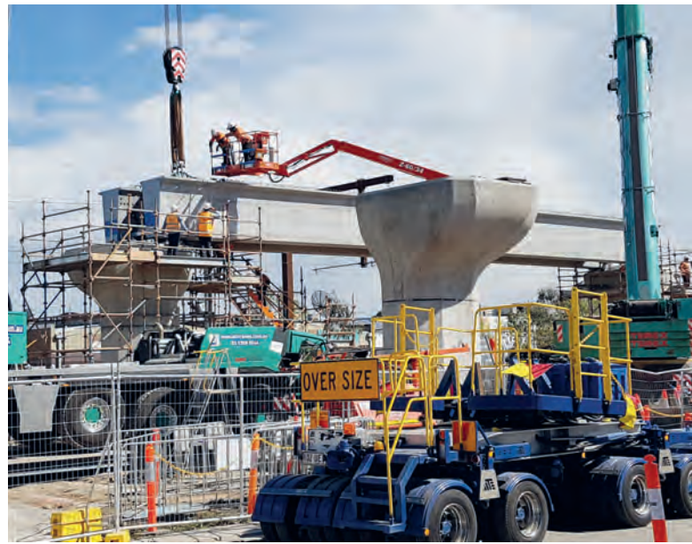
Installation of elements along the route
