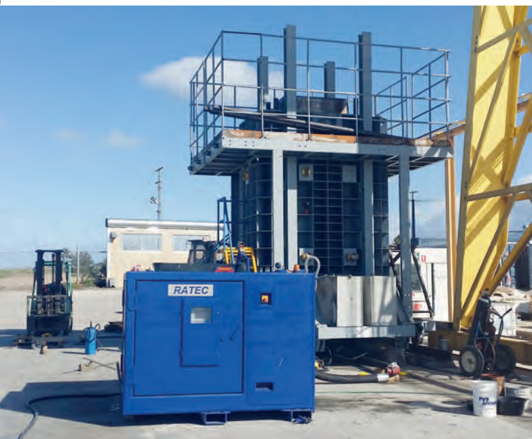
UPP100 and formwork for a support element
