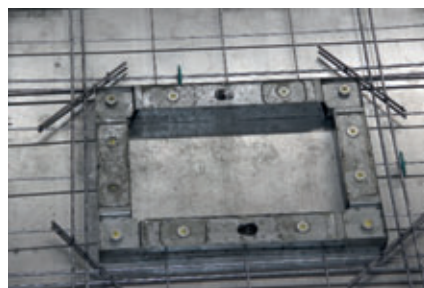
Recess based on the SAS formwork with 4 magnet holder edges
