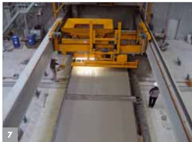
7 Concrete distributor with tandem scraper
