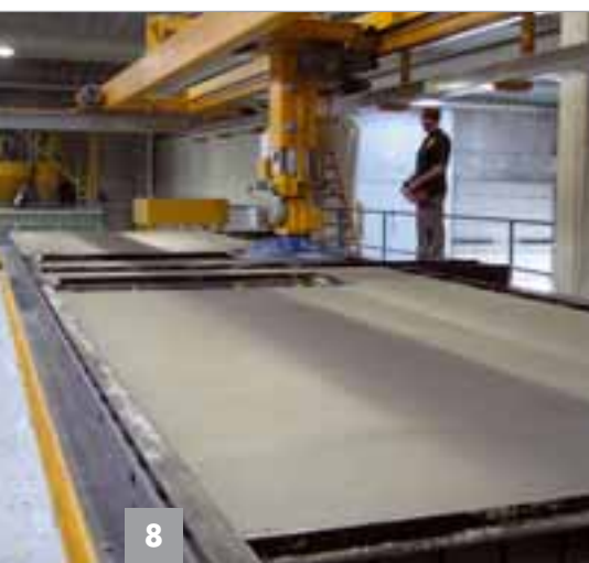
8 Smoothing of the concrete surface with radio-controlled smoothing equipment
