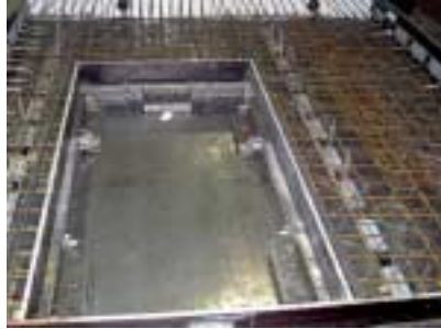
Fig. 3 Simple formwork solutions also for door and window openings.
