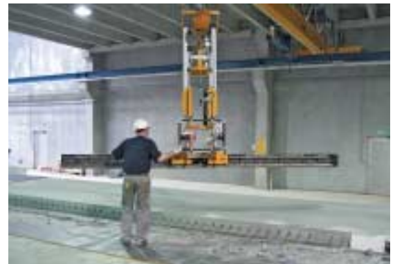
Fig. 2 Lifting of the formwork elements using the handling crossbar.
