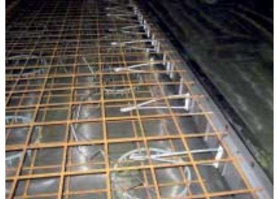
Fig. 5 Design of the casting groove with wire loop connection.
